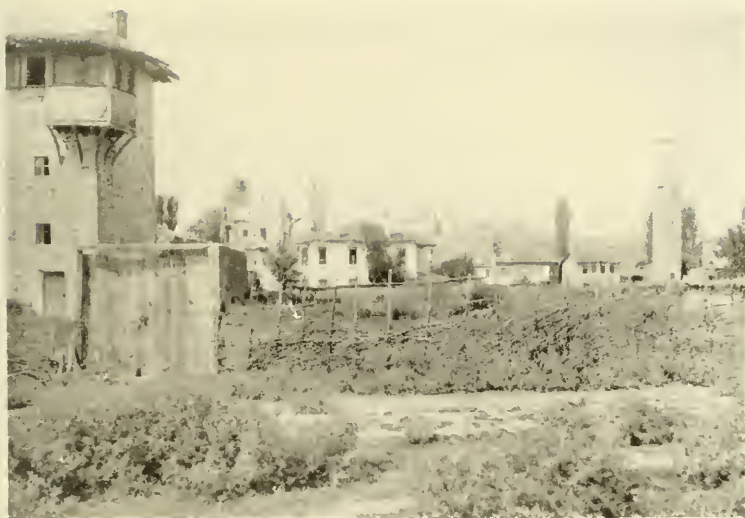
1. GHREVENA: CORNER TOWERS OF THE HOUSE OF MEHMED AGHA ON THE LEFT
