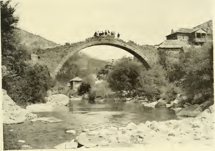
1. BAJEASA: BRIDGE OVER THE AOUS
